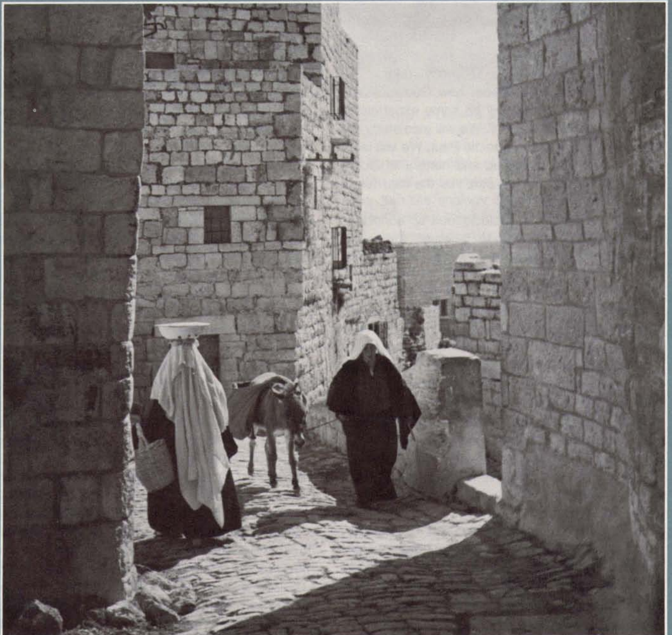
The New Testament Church
